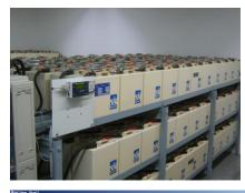
BLMG installation with a total of 540 batteries (6 V 150 Ah)
